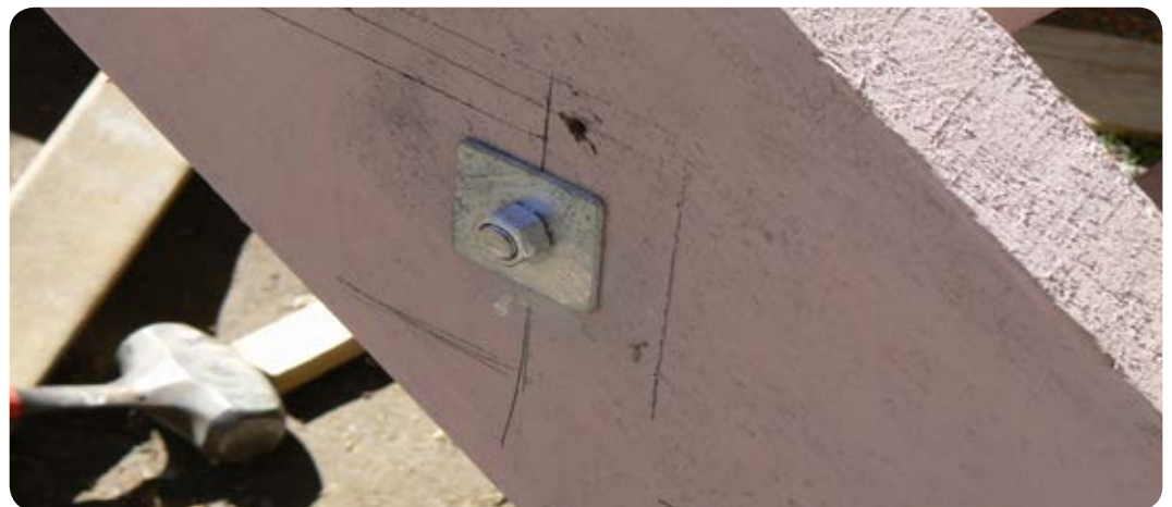
Figure 5.15: Position of step bolt.
