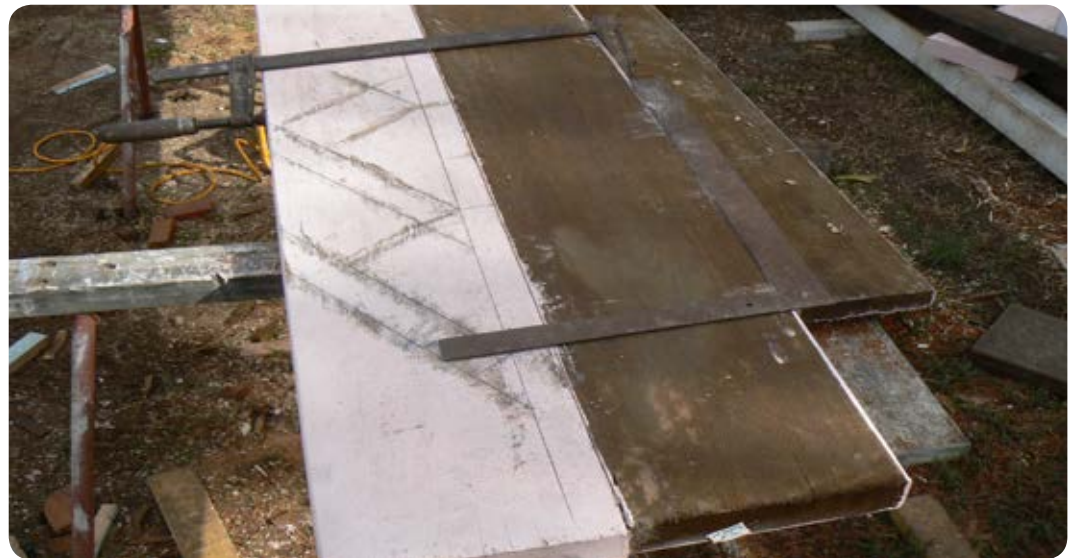
Figure 5.7: Marking out left string.
