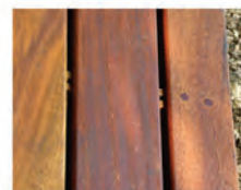
Installing the last deck board. Fasten the outside edge with surface screws, cover with plugs.
